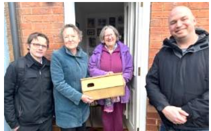
The installation of swift boxes
