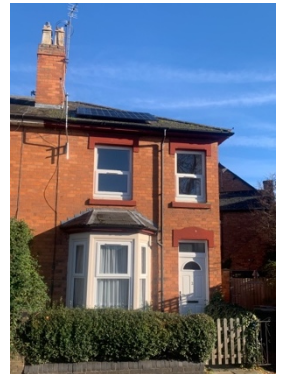
New doors, windows and solar panels on an older property in the Arboretum
